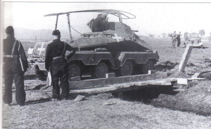
The heavier SdKfz 232 was widely used in German reconnaissance units. The cumbersome frame over the vehicle is for its radio antenna. The plain white Balkan cross was the standard German army insignia in the 1939 campaign. It was later replaced by a less conspicuous black cross with white outline as it proved too evident a target. (NARA)
