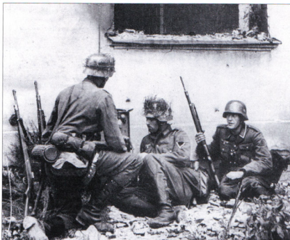
Radios proved important not only to the mobile forces but also to the infantry. This German infantry radio team is seen in operation during the fighting near Warsaw in September 1939. They are operating a Tornister Funkgerät d2 transmitter-receiver. Each infantry division had a radio company, divided into 21 radio sections, four with this particular type of set. (NARA)
